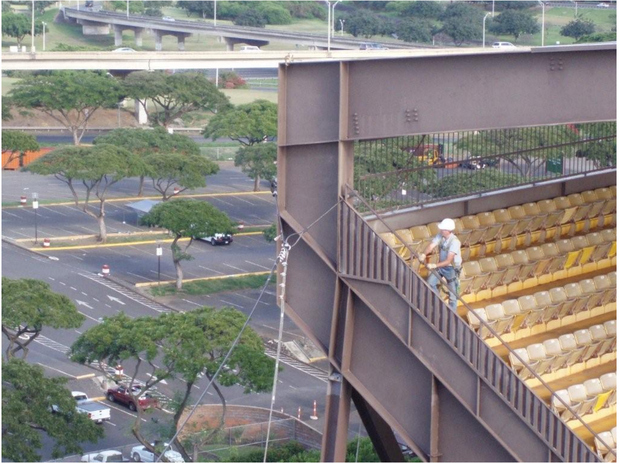
Cable Supported Platform Tie Back To Adjacent Girder
