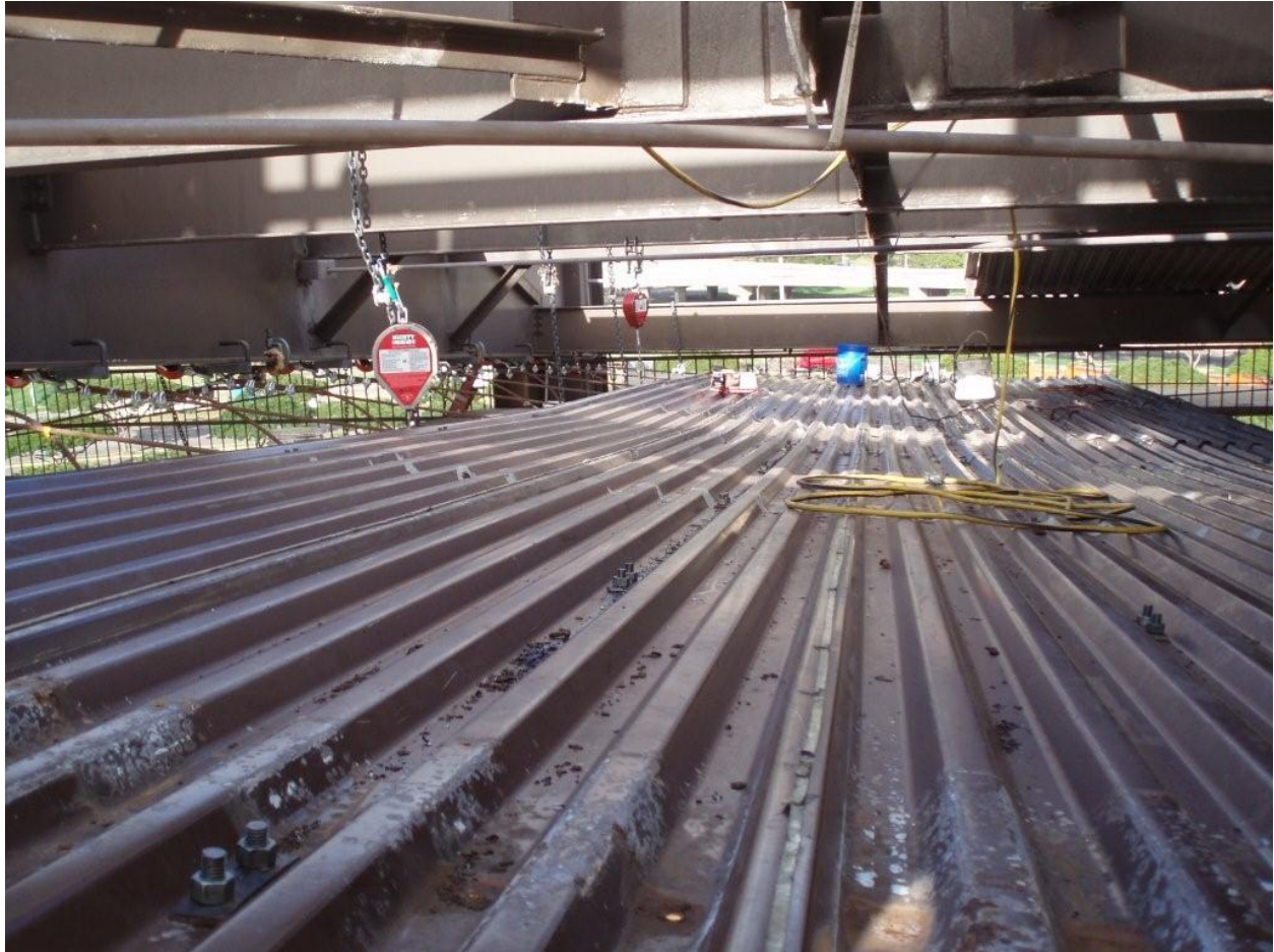
Cable Supported Platform – Below Upper Roof Deck
