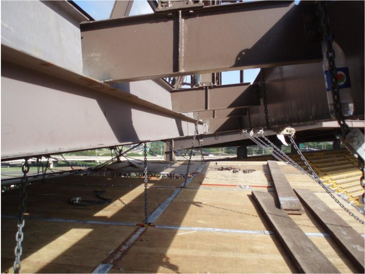
Quik Deck Platform – Below Upper Roof Deck
