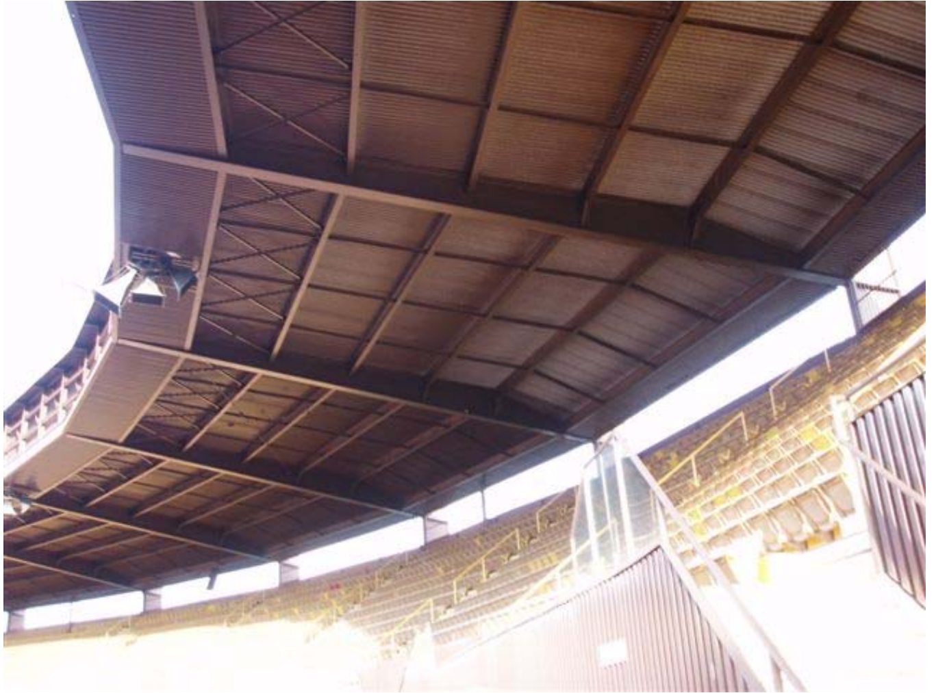
Upper Level Roof
