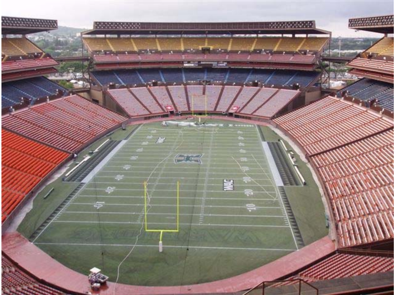
Aloha Stadium Roof Replacement Island of Kauai, Hawaii
