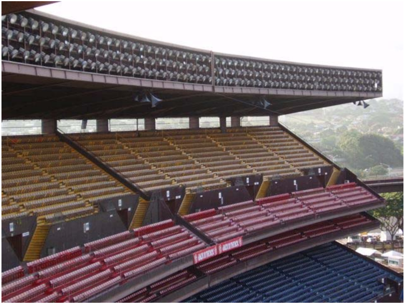
Upper Level Roof Area and Lighting
