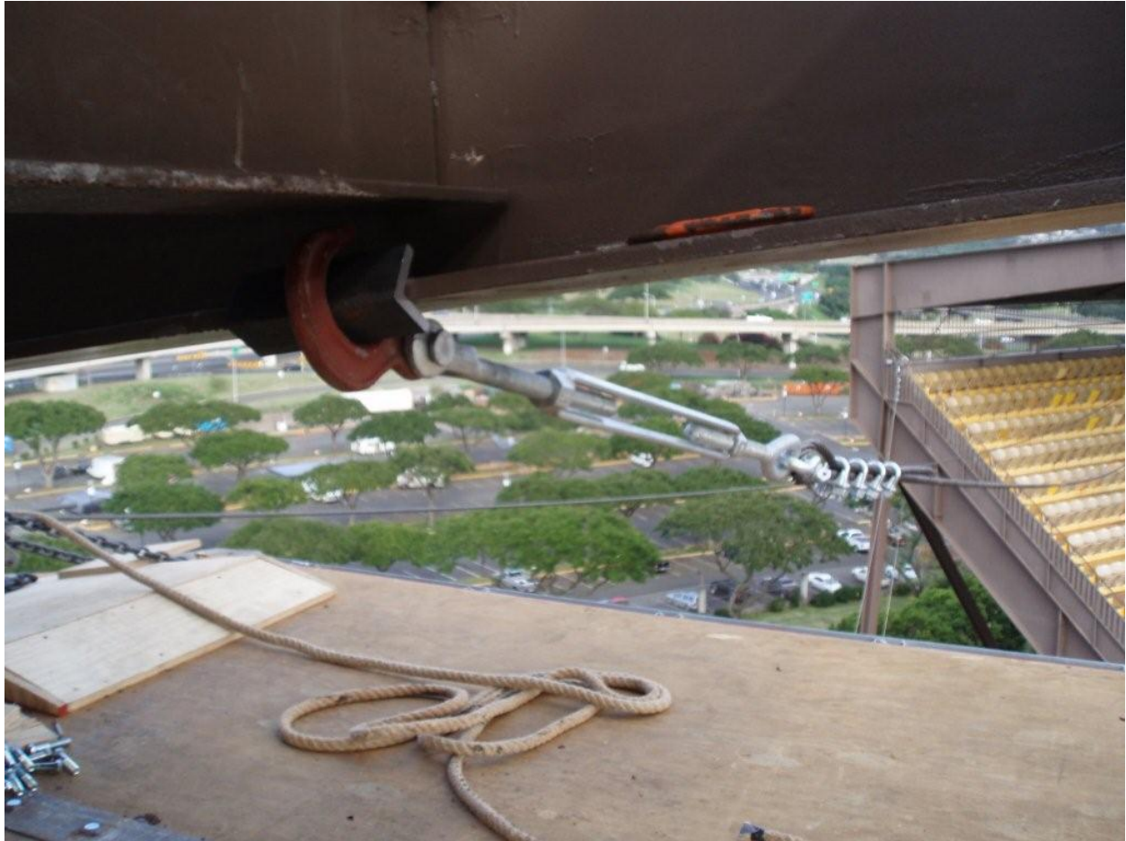
Cable Supported Platform Girder Tie Back Assembly
