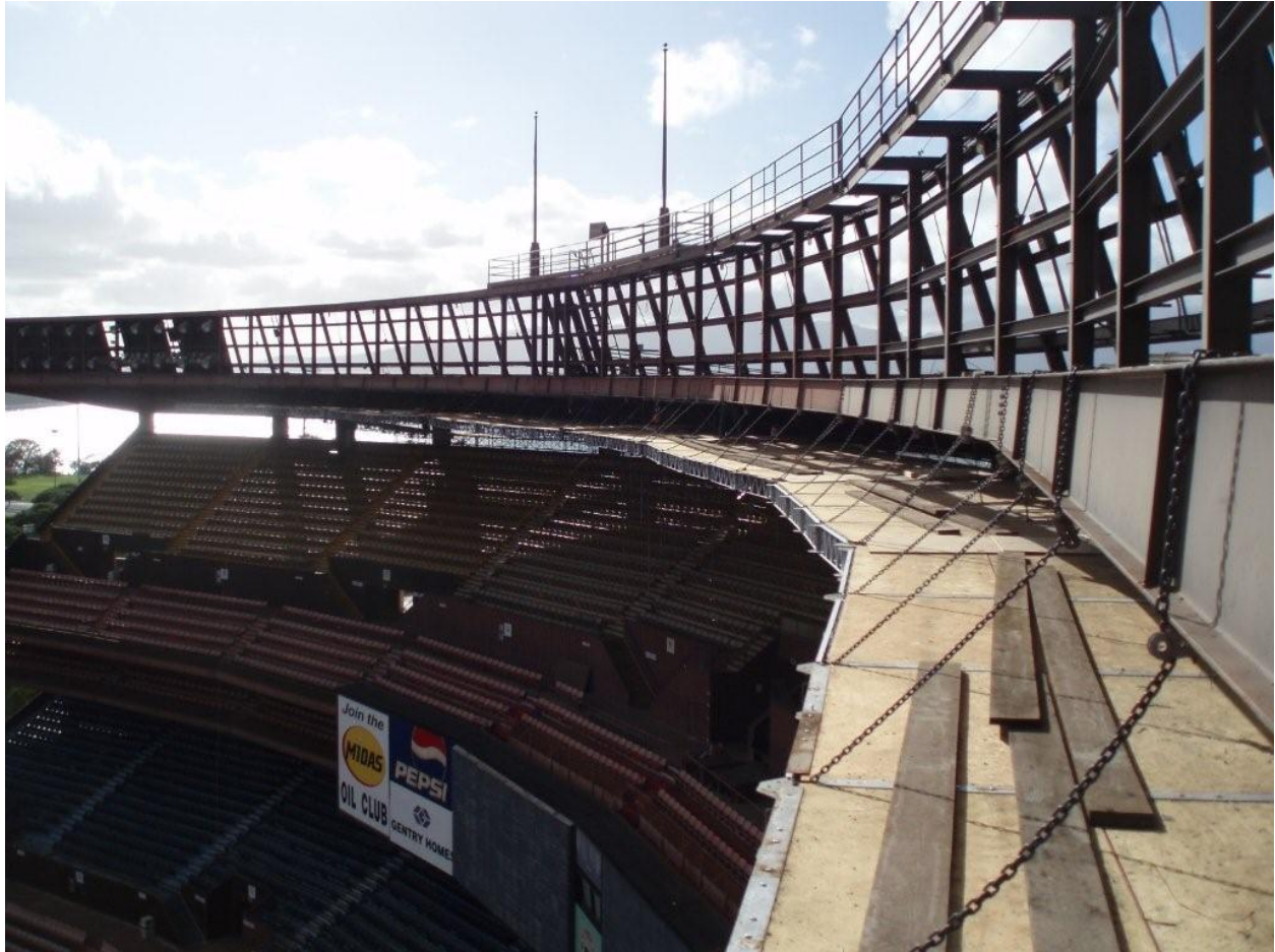
Quik-Deck Platform – Below Upper Roof Deck
