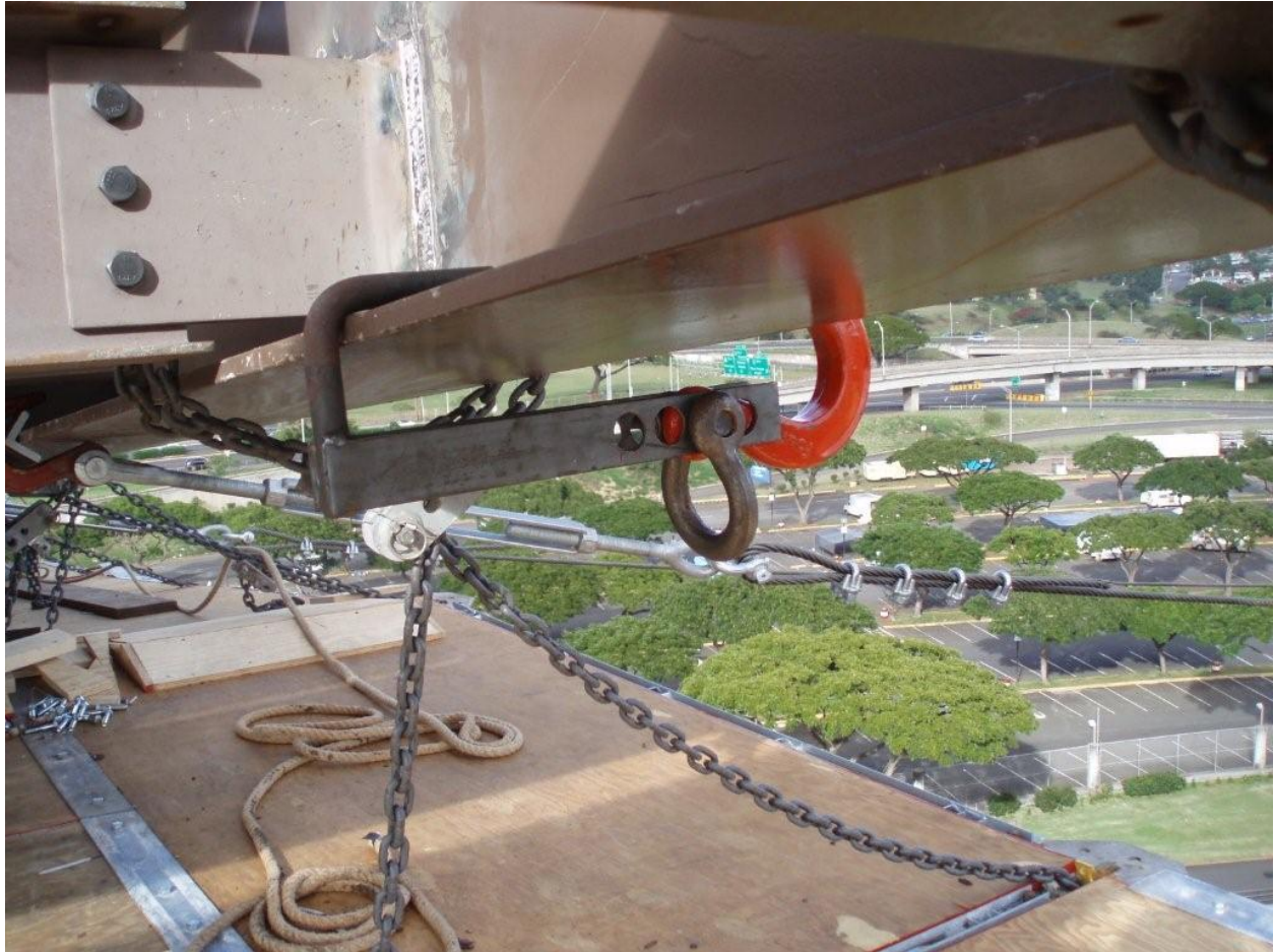
Cable Supported Platform Main Cable Hook To Floorbeam Support
