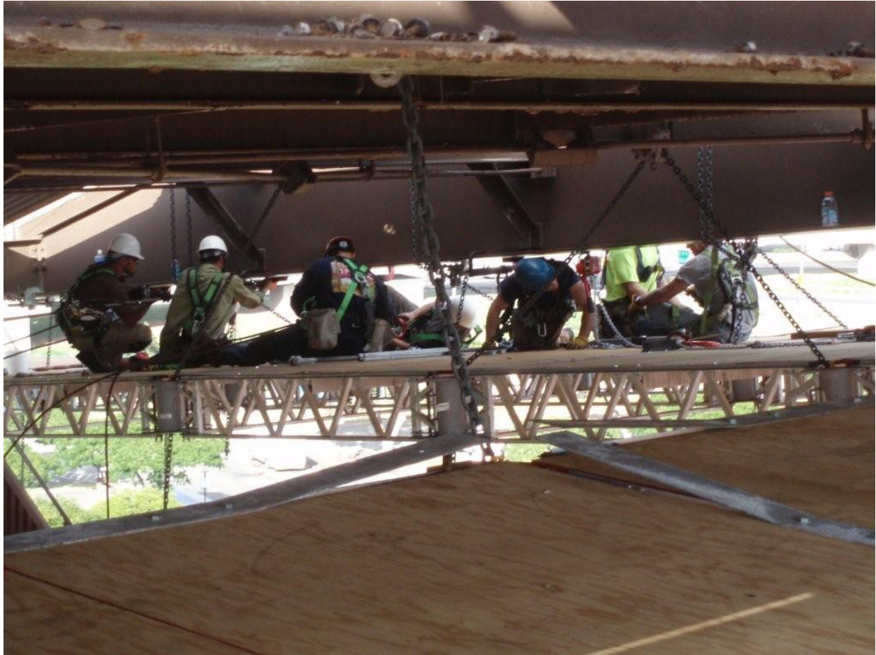
Quik Deck Platform – Below Upper Roof Deck
