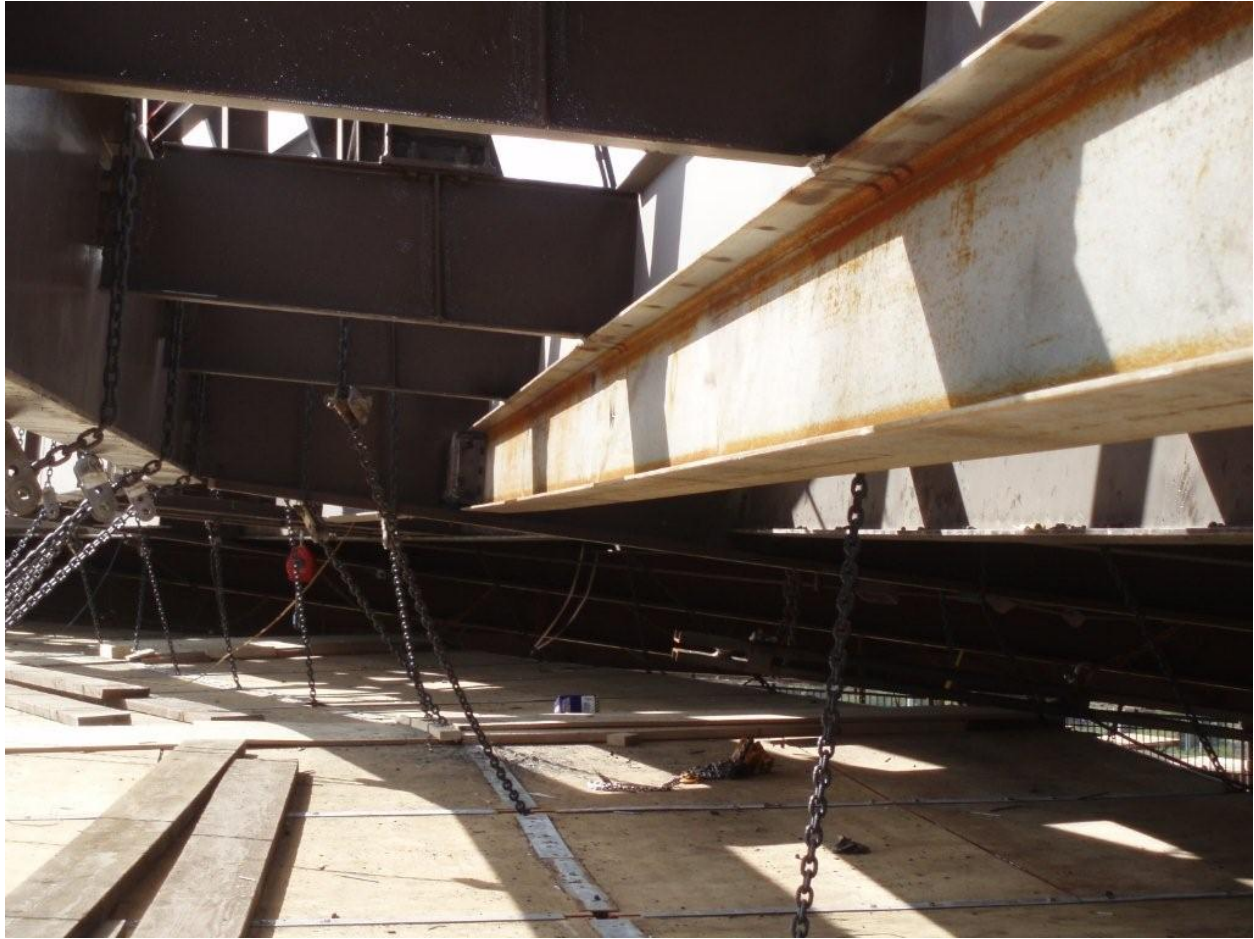
Quik Deck Platform – Below Upper Roof Deck
