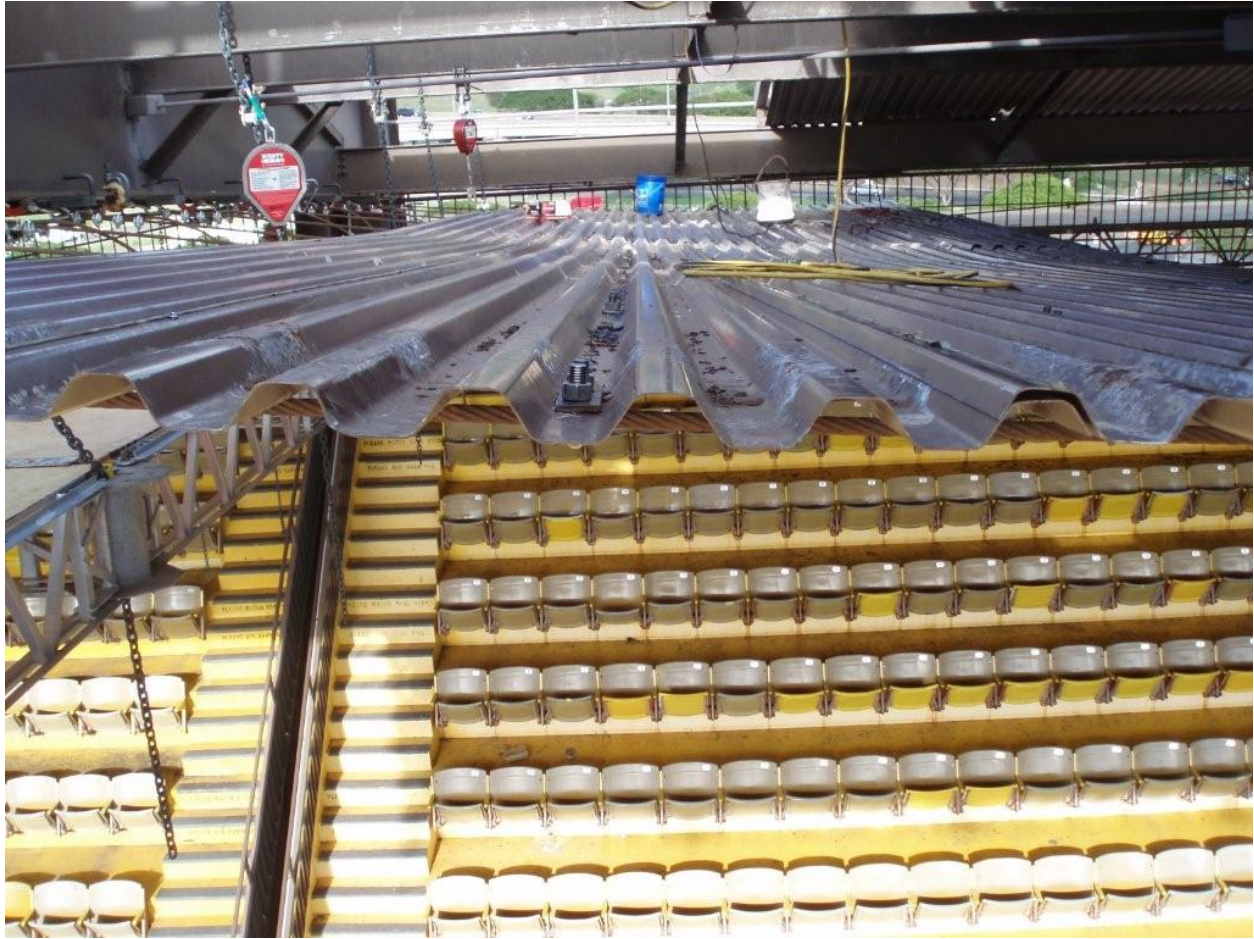
Cable Supported Platform – Below Upper Roof Deck
