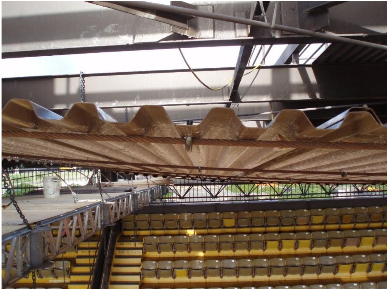
Cable Supported Platform & Quik Deck Platform – Below Upper Roof Deck
