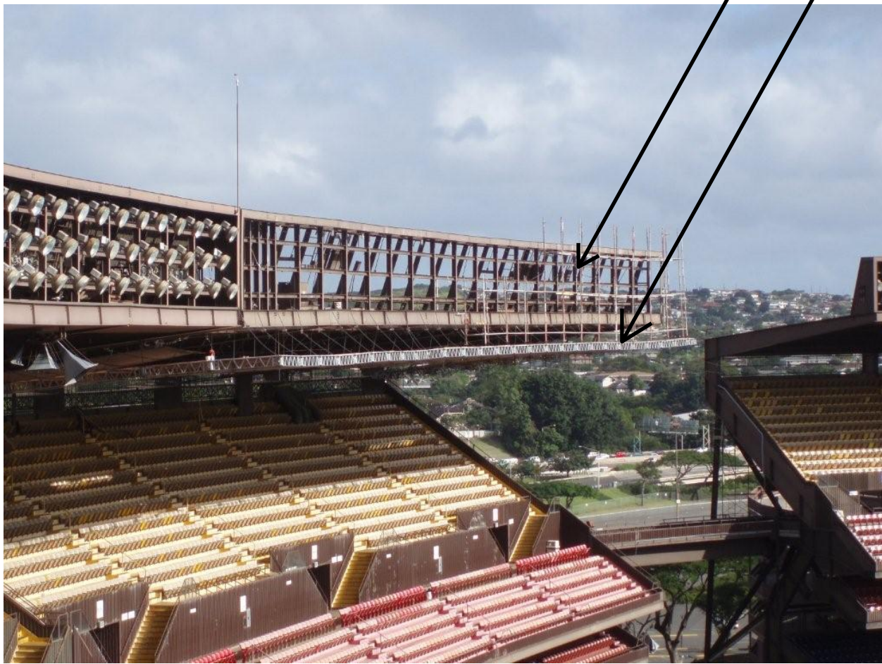
Quik-Deck Platform/Scaffolding – Below Upper Roof Deck
